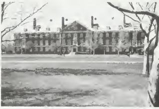
Unifying roof, David Kinley Hall
